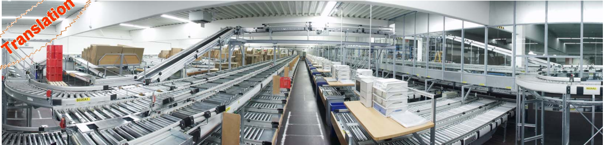
Distribution center for IT accessories: a permanent flow of goods and a high availability is prerequisite in the online-trade.
