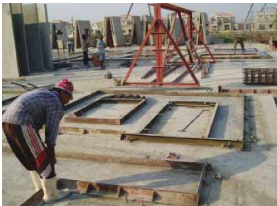
Casting Yard Preuksa
