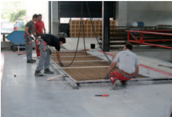
Inserting reinforcement at the next station
