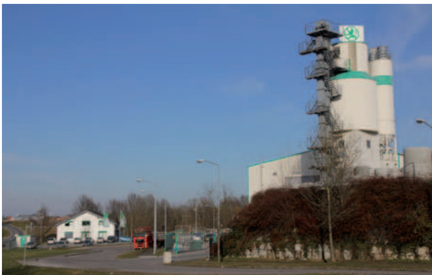
Penig production facilities of Heidelberger Betonelemente GmbH & Co. KG
